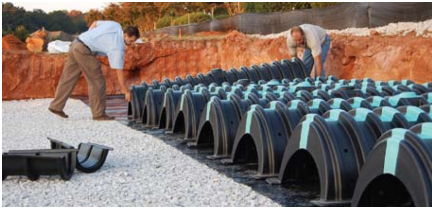
Runoff from the retail plaza is stored in the chambers, then piped into a drainage swale.
