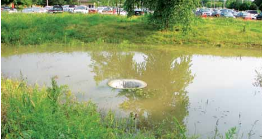
The filter intercepts the majority of the most frequently occurring runoff.
