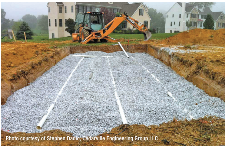
Left: This seepage bed in Chester County, Pa., allows rainwater to seep into the ground. Above: Water flows slowly through Longford Pond in Fitchburg, Wis., allowing more of it to seep into the soil.
