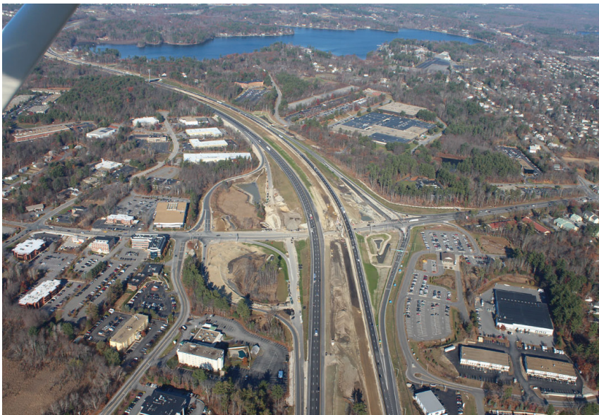
The $795 million I-93 project will add an additional two travel lanes in each direction over the entire 20-mile-long road. Storm water collection systems gather runoff all along the road.
