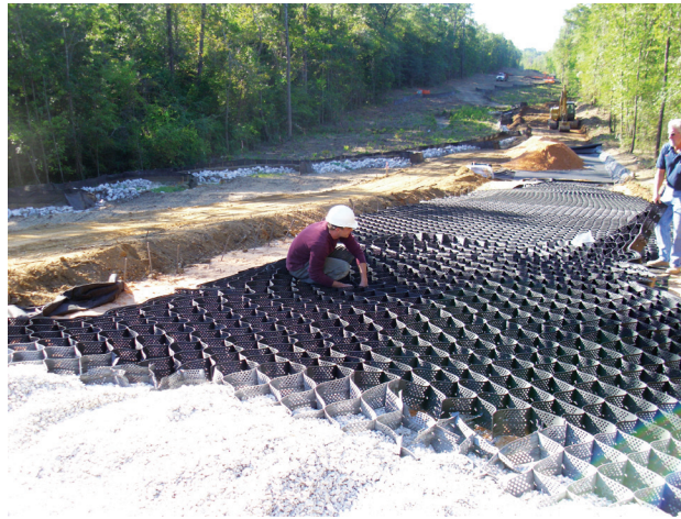
The geocellular system stabilizes the aggregate, preventing movement under vehicle load, and also allows storm water to drain into the soil rather than run off.
