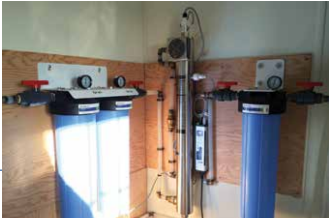
Rainwater is made potable with sediment filtration, ultraviolet disinfection and carbon filtration.
