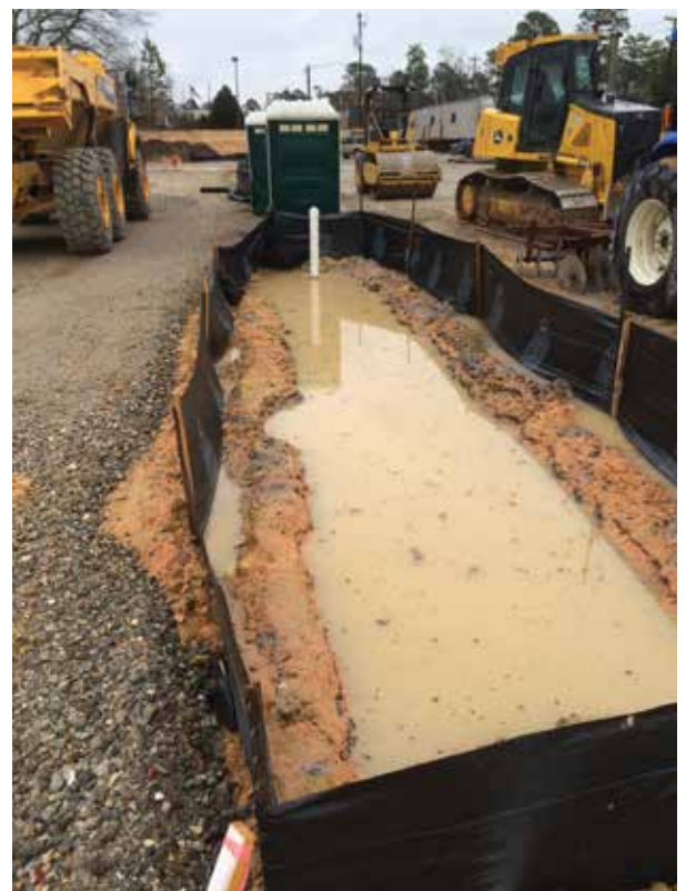
Top left: A rendering of a typical bioretention cell at maturity. Bottom left: The finished basins include crosswalks for customers and salespeople. Right: A bioretention basin built out of the recommended sequence. The basins built out of sequence had to be rebuilt due to sediment contamination.
