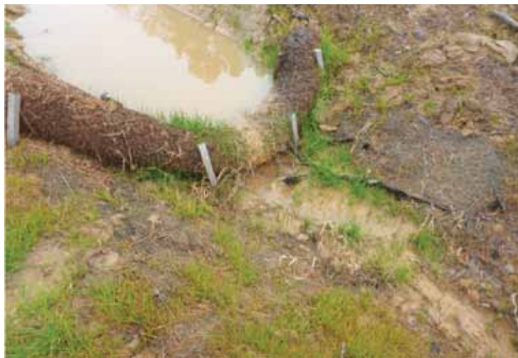
Fiber check dam and granular polyacrylamide applied at a construction site.
