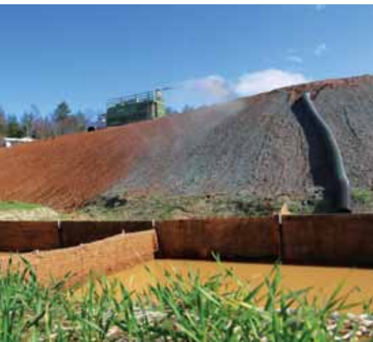
The hydromulcher allows the crew to spray up to 2 tons of limestone, 500 lb of fertilizer, 150 lb of grass seed mix and 400 lb of mulch in one application.
