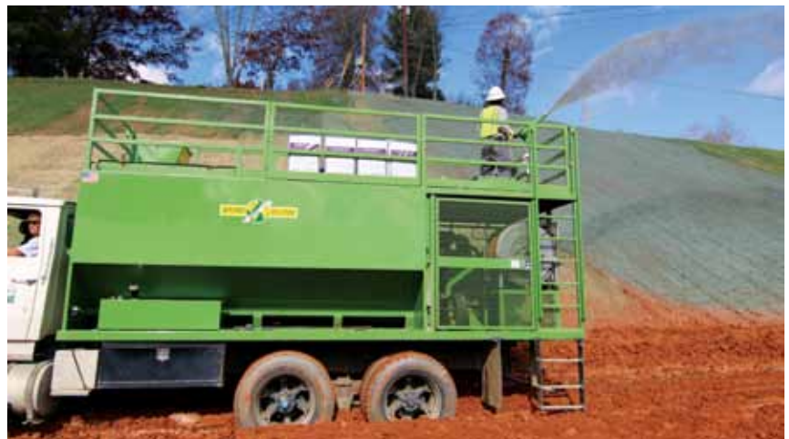
The hydromulcher allows the crew to spray up to 2 tons of limestone, 500 lb of fertilizer, 150 lb of grass seed mix and 400 lb of mulch in one application.
