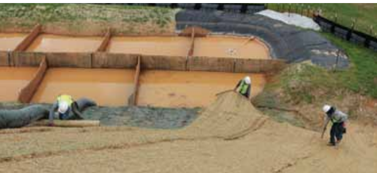
Double-net straw matting is used on almost all NCDOT projects.
