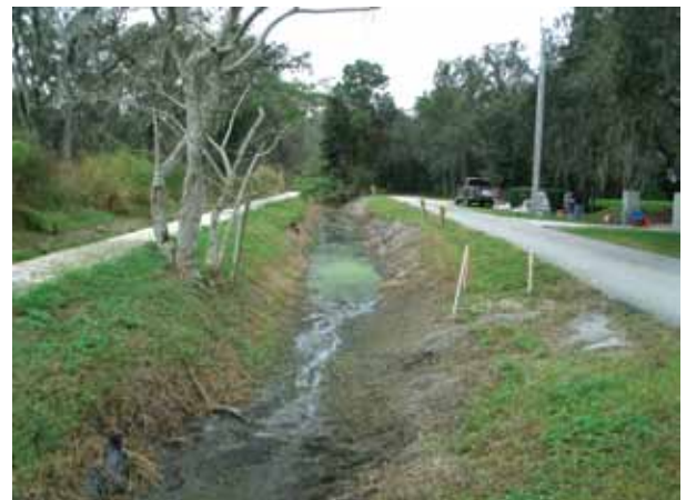
The underdrain/exfiltration system (right) functions as a wet detention pond and provides modest water quality pretreatment for the contributing basin area prior to discharge to the receiving canal system.
