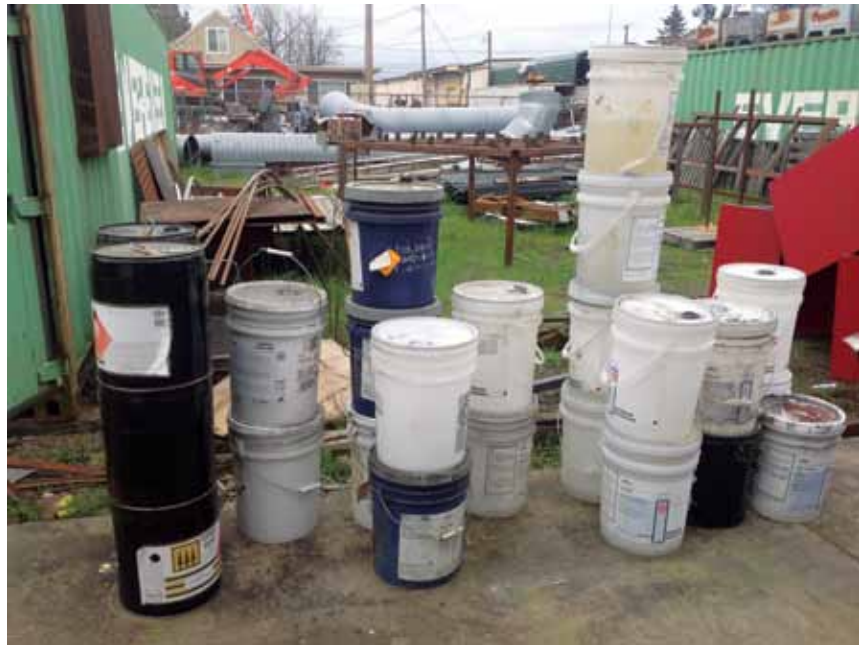
An example of improper storage of hazardous materials, a possible permit violation.
