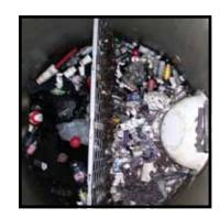
The Beacon Bluff installation was monitored from Oct. 14, 2011, through Sept. 28, 2012. More than 130 cu ft of sediment were removed. Floatables removals were observed and estimated at above 85%, with several cubic yards of floatable trash and debris being removed. More than 65,000 Snouts and more than 700 SAFL baffles have been installed in North America.
