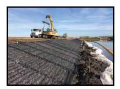
$114\,\mathrm{mattresses}$  (7,463 sq ft) off site, filling the mattresses with AASHTO 1 stone (1 to 4 in.). While the majority of the mattresses were rectangular and 10 to 15 ft in length, GeoSyn specially fabricated two trapezoidal mattresses to accommodate irregular formations at the site. Once delivered, the mattresses were lifted directly from the trucks and set in place by a six-person crew from Ritacco Construction Inc.
