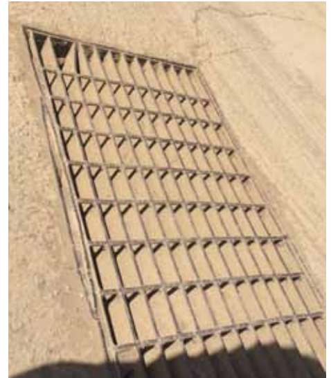
Here, a good housekeeping BMP (sweeping) has not been effective, so a sediment control BMP (a drain inlet filter) is likely necessary.
