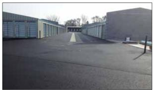
The permeable pavement was designed to capture and retain the water from all runoff events up to the 100-year design storm (4.4 in. of runoff).
