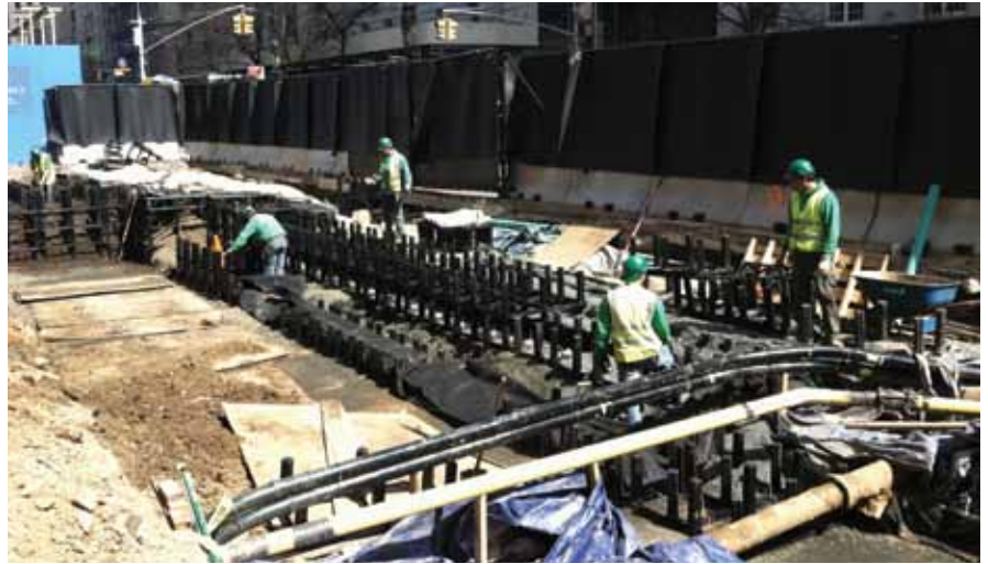
The water is filtered by varying dimensions of bioretention media, depending on system depth, and then enters the overflow pipe at the bottom of the system—cleaner, cooler, slower and in lesser amounts due to bioremediation.
