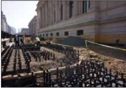
The water is filtered by varying dimensions of bioretention media, depending on system depth, and then enters the overflow pipe at the bottom of the system—cleaner, cooler, slower and in lesser amounts due to bioremediation.
