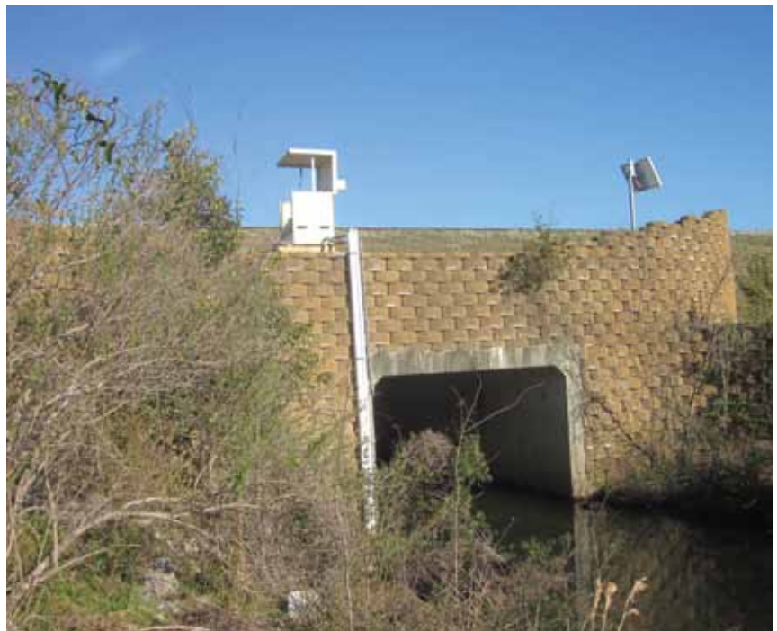
MCAS had five permitted storm water outfalls that needed monitoring instrumentation.
