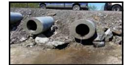
last culvert was a 36-in. round 40-ft CMP that was relined with a 28-in. pipe.
