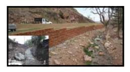
ity wall consists of 28- and 60-in. blocks in the Ledgestone texture. The wall reaches heights of about 12 ft and is engineered to withstand future flooding.
