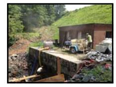
and installing a sandbag and poly sheet cofferdam to hold back water for about five hours.
