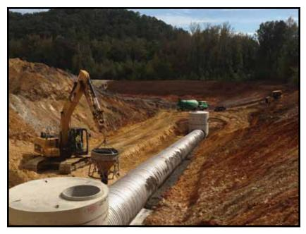
weight of the ALT2 spiral rib pipe. Andy Cook of John D. Stephens said, "Given Contech's capability of making the pipe joints in 40-ft lengths, our laying time for each joint decreased by almost 30% and provided a substantial cost savings to the owner over the use of [another material]."
