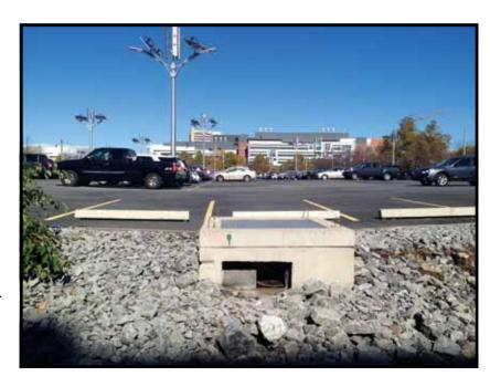
several benefits. Using the Jellyfish Filter to pretreat bioretention on a site with limited available drop makes the flexibly designed filter a good fit. The unit's placement—along the curb line with a hatch—provides a single point of access for easy inspection and maintenance.
