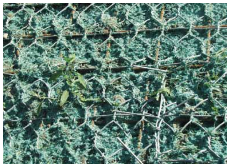
A biotic soil amendment was applied to the exterior of the system.
