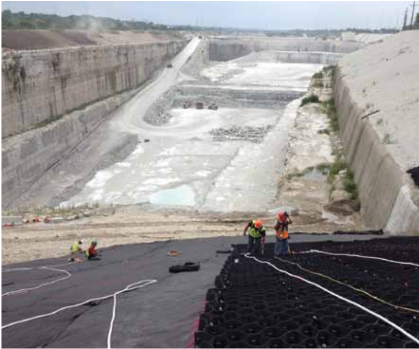
The system with aggregate and concrete infill provided a flexible, hard-armored, long-term slope cover.
