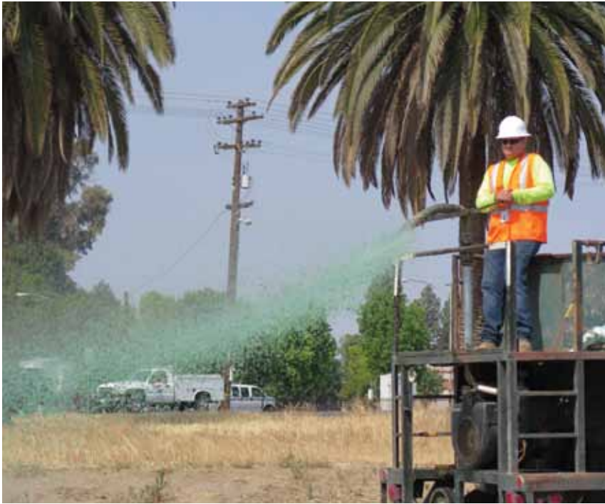
The product can provide immediate dust and erosion control and soil stabilization until permanent vegetation is established or construction has resumed.
