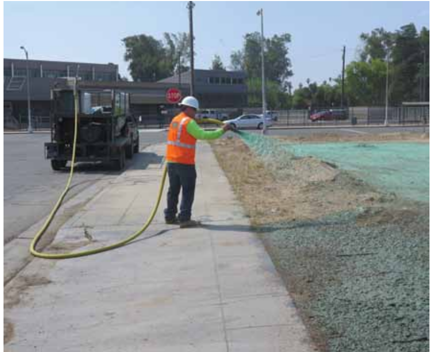
The product is designed to work directly with soil to maintain its stability, both by preserving existing soil structure and flocculating fine sediment dislodged by storm water or wind.
