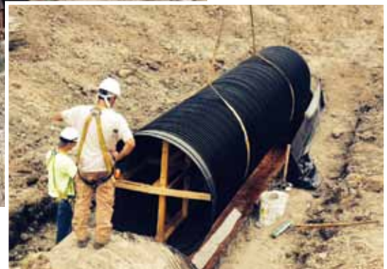
Use of conventional round liner pipe would have required considerable downsizing in order to provide adequate clearance during the installation process.
