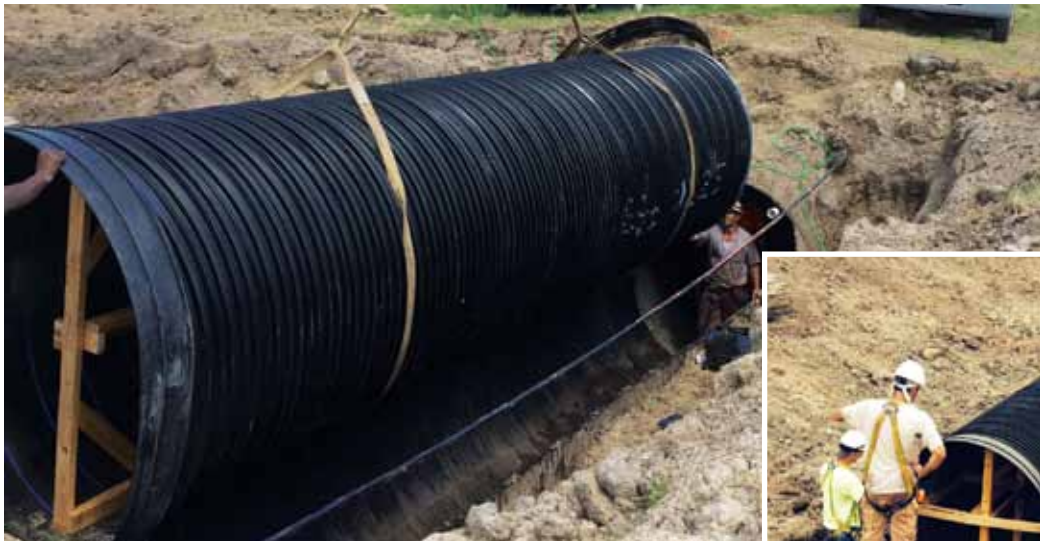
Use of conventional round liner pipe would have required considerable downsizing in order to provide adequate clearance during the installation process.
