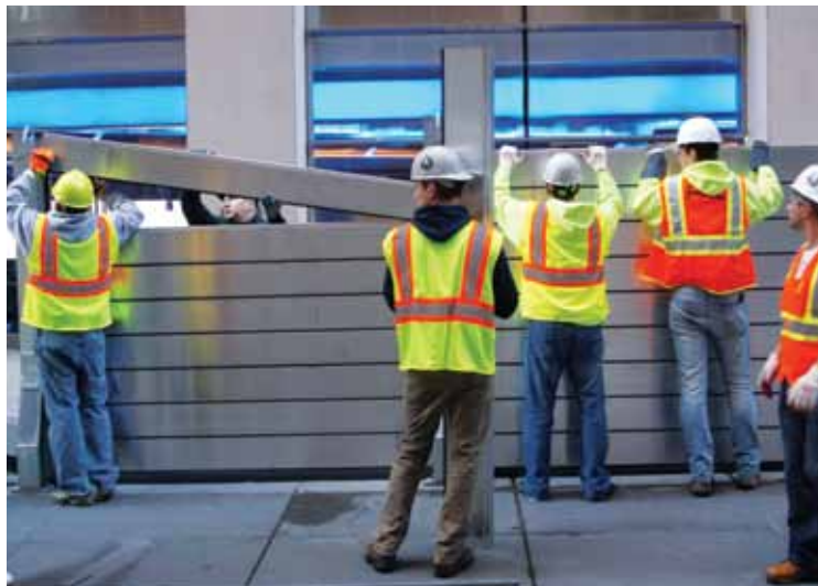
Each barrier for 55 Water Street called for customization because of how weather affects the building at each angle due to the surrounding rivers.
