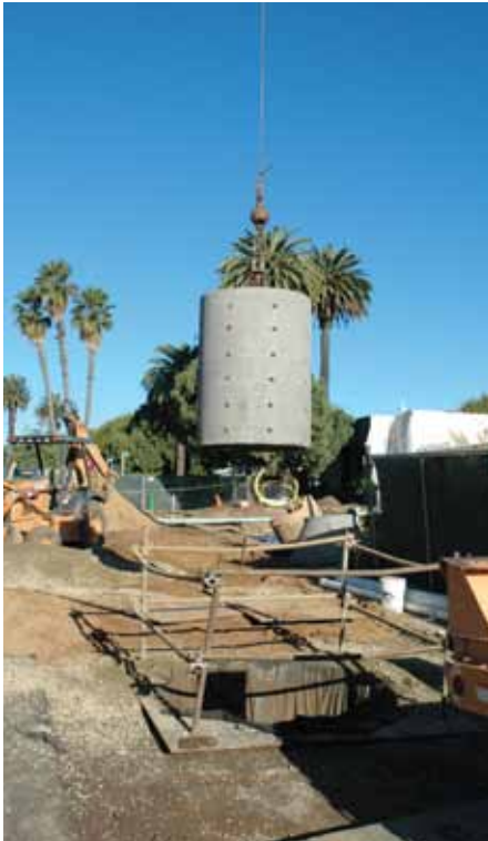
The rainwater storage tank is lowered into place.
