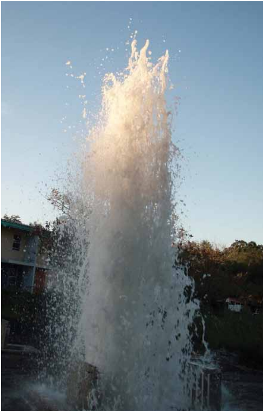
Geysering drainage wells are of particular concern because they usually are in urban settings where the violent discharge of water can become a threat to public health, safety and welfare.
