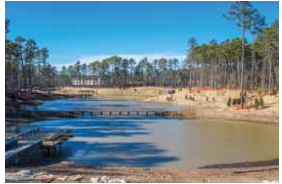
The boardwalk and pavilion decking for the project are constructed of wood from trees harvested and processed during clearing of the site.
