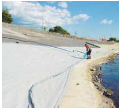
Engineers dewatered the reservoir and installed a seamless spray-on polyurea liner over geotextile fabric to create a watertight membrane.
