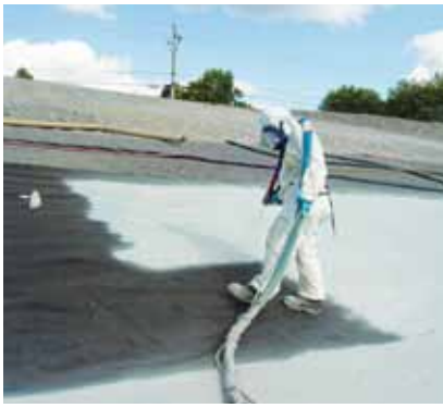
Engineers dewatered the reservoir and installed a seamless spray-on polyurea liner over geotextile fabric to create a watertight membrane.
