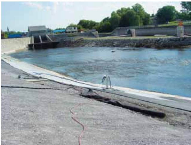
The McLeod Dam in Ontario, Canada, is a hydropower facility that powers the equivalent of 400 homes.
