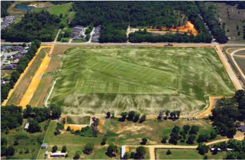
An aerial view of the Saufley Field disposal site near the Saufley Field Navy Air Base in Florida
