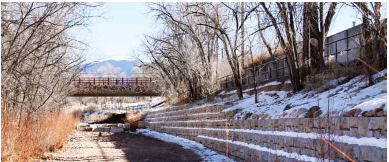
As the population of Santa Fe has grown, runoff has increased, eroding the Santa Fe River bed.
