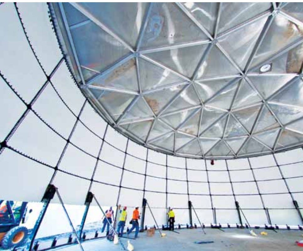
A wastewater storage tank is constructed.
