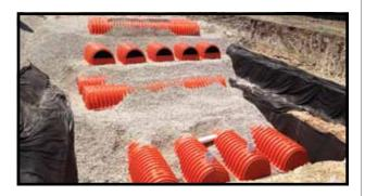
possible only because the system is capable of supporting more than four times the H-20 wheel load rating (more than 32,000 lb per sq ft), as documented by independent laboratory testing. The system was able to accommodate the required 25,000 cu ft of storage within a 126-by-33-ft area (4,158 sq ft total).
