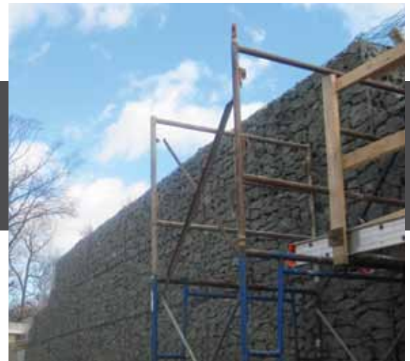
When gabions are filled with stone, they become large, flexible building blocks from which a broad range of structures can be built.
