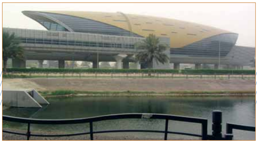
A drainage pond located on the Mall of the Emirates grounds
