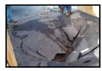
unstable soil surrounding the pipe, so to prevent similar problems for the rehabilitated culvert, Clayton County Water Authority (CCWA) stabilized the surrounding soil with cementitious grout, injected until refusal.
