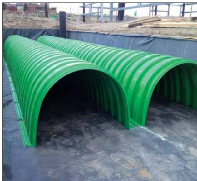
The chambers will harvest rainwater that will support a plant nursery and local firefighting needs.
