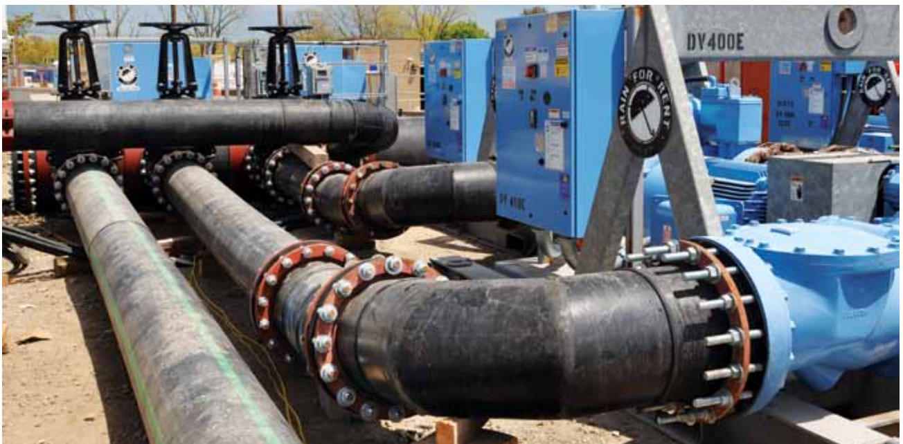
The bypass system setup
