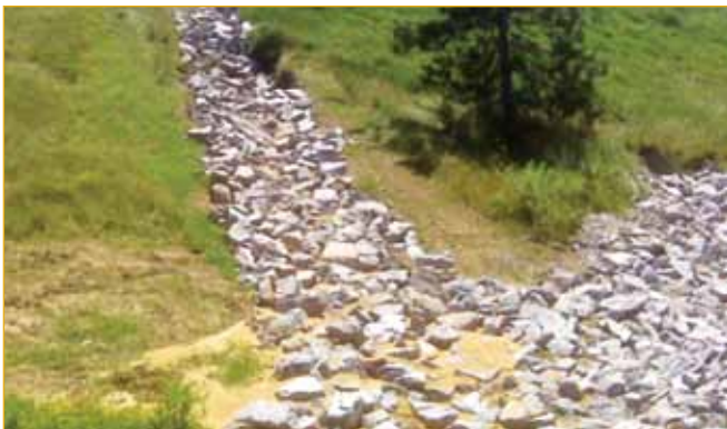
Riprap was used for steep drainage outfalls on a highway overpass.
