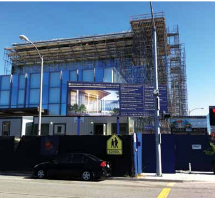
The new Gov. George Deukmejian Courthouse, mid-construction
