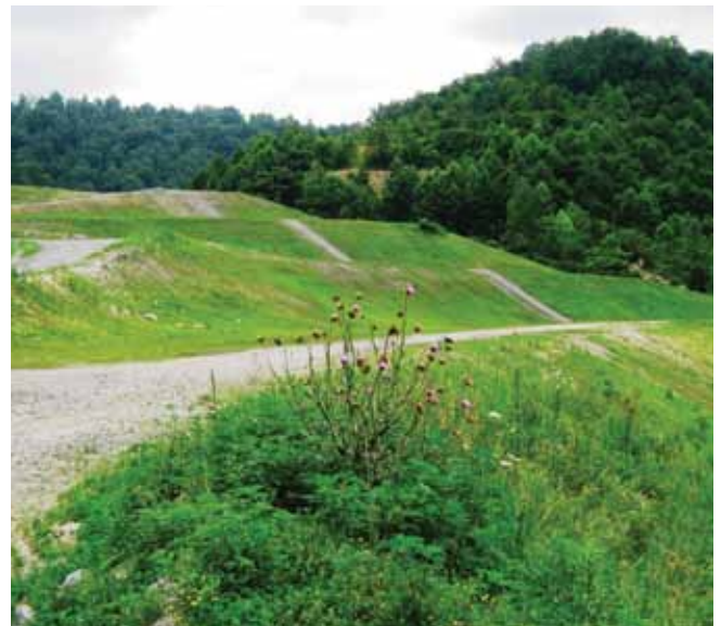
Left: The slopes went through a process of shaping and preparation before seeding. Right: The seed was hydraulically applied along the slopes and vegetation was quickly established.
