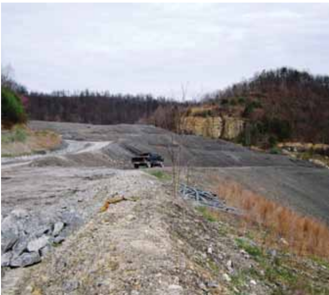
Left: The slopes went through a process of shaping and preparation before seeding. Right: The seed was hydraulically applied along the slopes and vegetation was quickly established.
