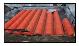
SedimenTrap. Soleno was able to make the school board aware that plastic storm water chambers are not restricted to use for infiltration purposes. The company designed a StormChamber system lined with an impermeable geomembrane that would prevent backflows from leaching into the ground. The system solved the school board's problem and made it possible to achieve the cost savings of a plastic storm water system. SWS
