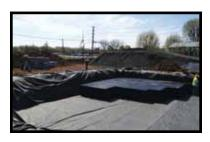
constraints, the designers decided to utilize Brentwood's single-stacked StormTank system. The basin provided an ideal solution to the problem by allowing slightly more than 10,476 cu ft of storm water storage, in addition to preserving developable land.
