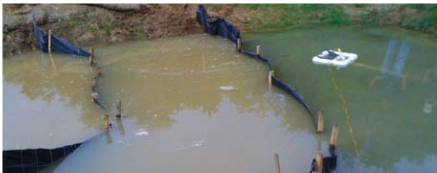
Initial results show that the TRSB system is successful in reducing turbidity to an acceptable level.
