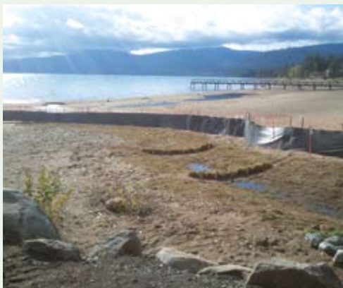
Mitigating historic watershed impacts at Kings Beach involved propagated wetland mats for channel stabilization.
