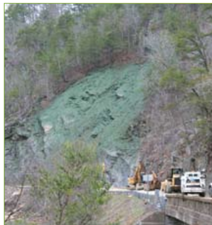
Workers hydromulched the 250-ft, 1:1 slope, resulting in significant vegetation growth.
