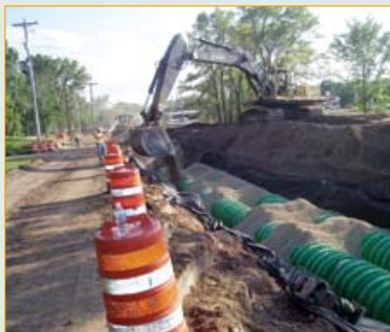
Three separate infiltration systems provide the city the storage volume capacity it needs to comply with regulations.
