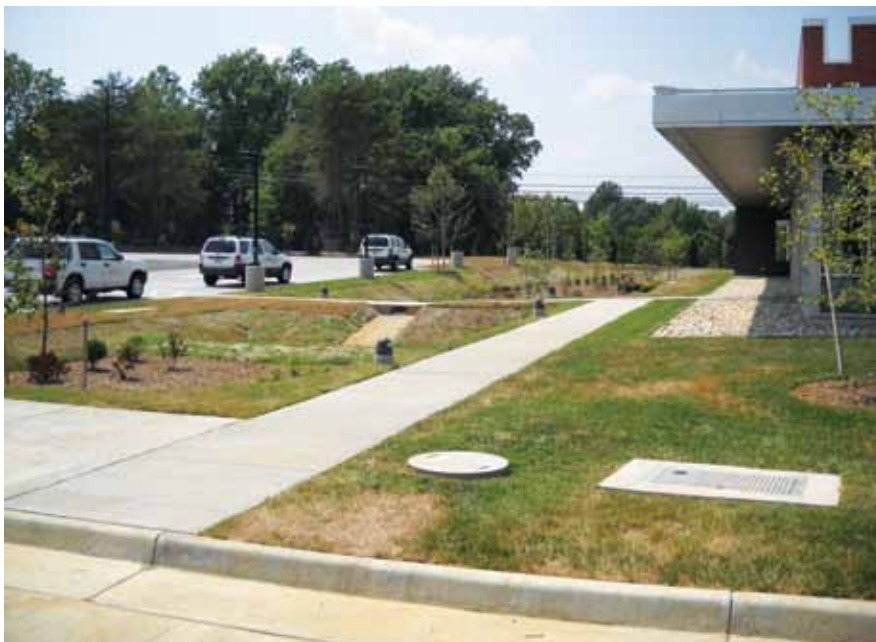
The rain gardens located to the south of the facility were positioned to create a focal point at the entrance used by the facility's staff and bus drivers.
